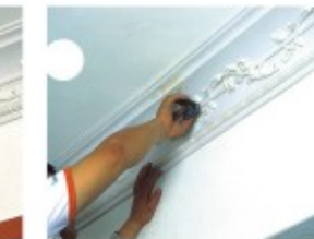
10. Allow to dry, sand smooth with sanding paper and finished with paint.
