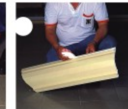
4. Apply construction glue to contact points of cornice to wall and ceiling.
