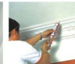
8. Apply filler (silicone & plaster) to fill up gaps.
