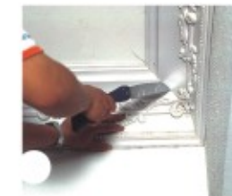
6. The joints between the cornice can be amended with the sanding paper.
