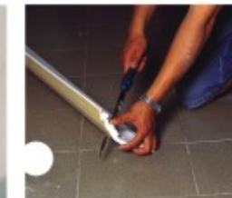
3. Saw at the marked point of the cornice, and better to cut more than 5mm.
