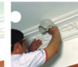
9. Cleaning overflowed glue with the waterish cloth.
